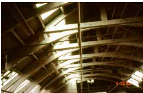
Figure 23 Laminated beams without glue Halifax, UK, 1900
