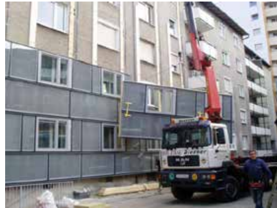
Figure 5 Preparation of SCIMFS units and attaching them to the existing wall [10]
